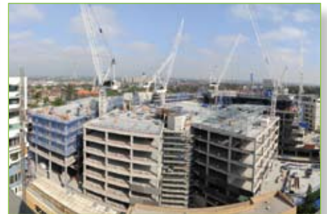
The construction site in November 2009.
